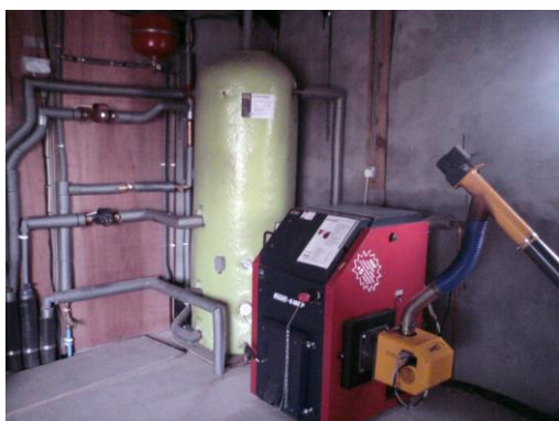
Kalvis 6MPP pellet boiler c/w 500 litre Thermal storage cylinder.
